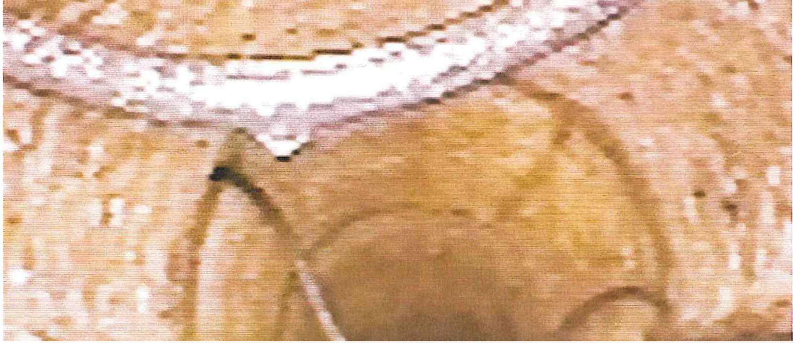
Current Condition of Collection System Structural Deterioration
